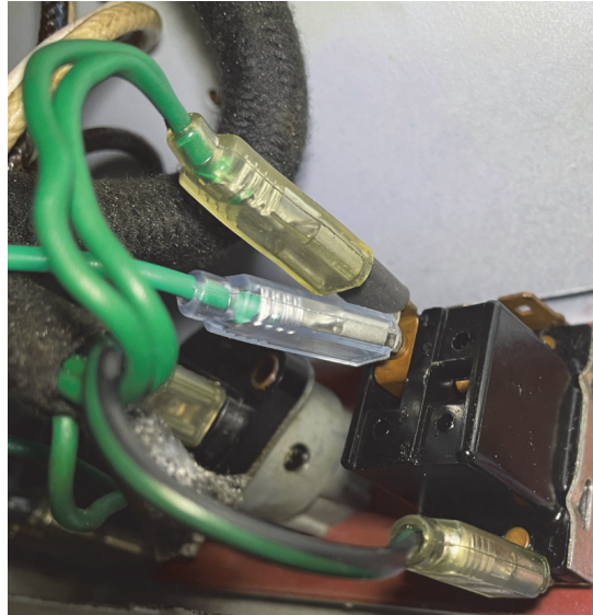
Fig. 9 Feed wires at the wiper switch using piggy-back connector.
