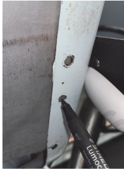
Fig. 3 Marking out holes in the switch panel shield
